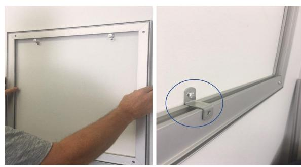
Clips installed across top of frame
