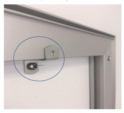
Metal Clips supplied with wall mount screws to secure frame to drywall as shown here:
