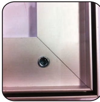
Connect profiles together and tighten lock. Image above shows a good connection.
