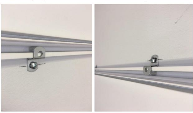
Clips installed across top of frame
